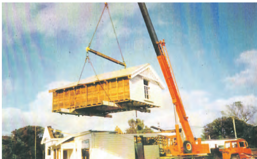
The attic being removed from the Morrieson homestead in 1993.
